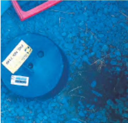
View looking into pit with Flood-Gate and cleanout with gravel ballast.
